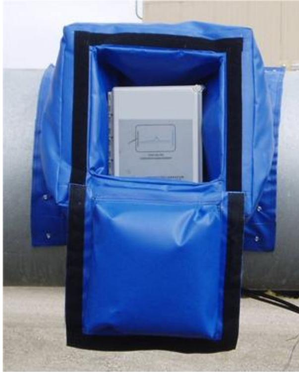
**Figure 6 - Insulating Enclosure**
