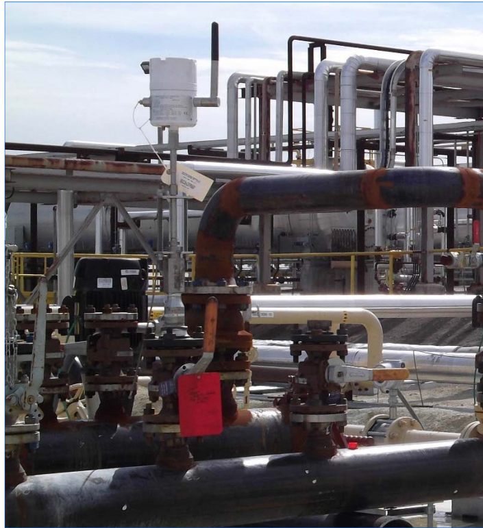
Microcor ER Wireless Transmitter and Low Pressure Probe Flange Mounted
