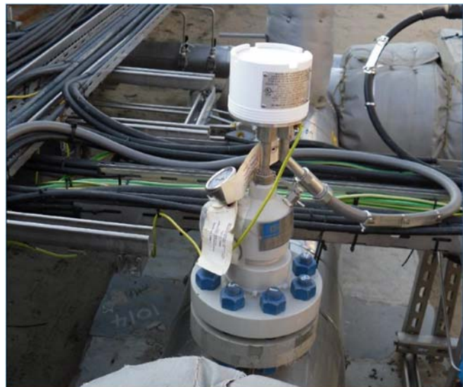
Microcor ER Transmitter and Probe mounted on a Cosasco High Pressure Flanged Access Fitting
