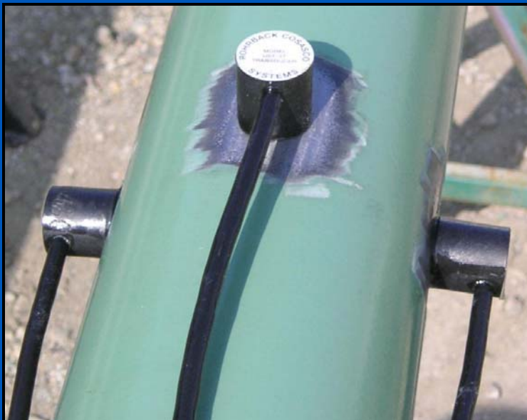
Sensors permanently bonded using epoxy to pipeline before installation
