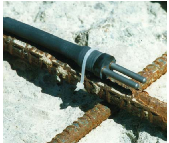
Probe mounted above the rebar Electrode length 1.25" (32mm)
