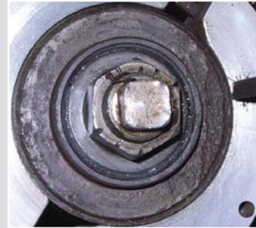
Access Fitting before re-facing
